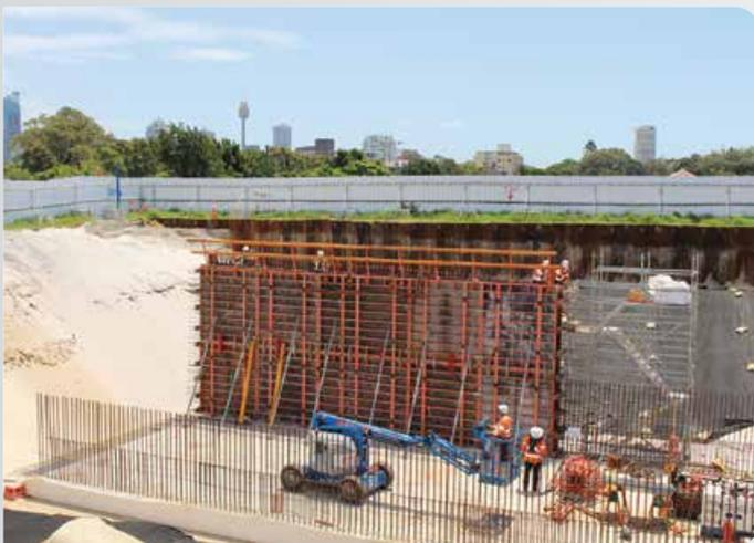
**3** Walls were installed in eight sections.
