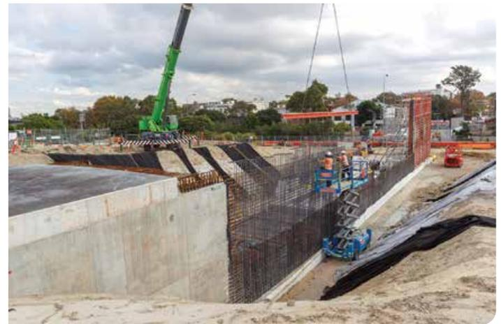
**8** Work is currently underway to build the portal that will connect the tunnel to the Eastern Distributor bridge.
