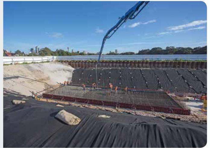
**2** The concrete base slab of the tunnel was installed in three sections.
