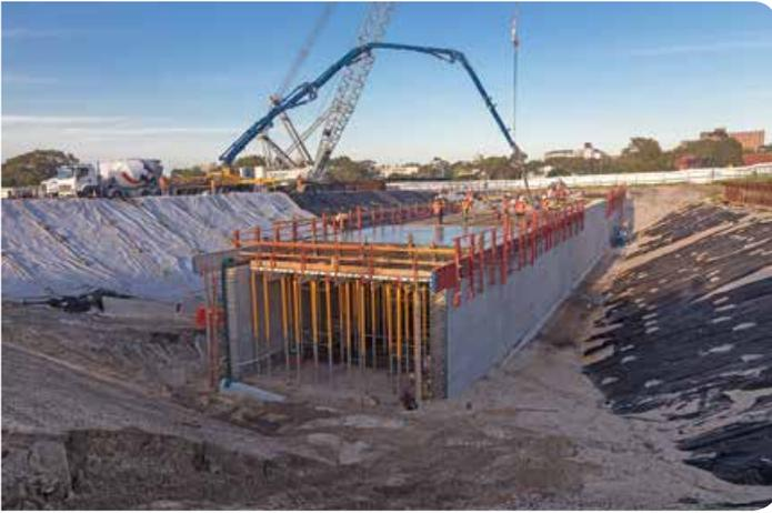
**5** With the walls in place, a framework was installed to support the concrete roof installation.
