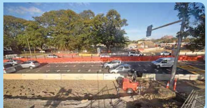
permanent pedestrian and cycle path in place, excavation of the tunnel under the roadway is underway.
