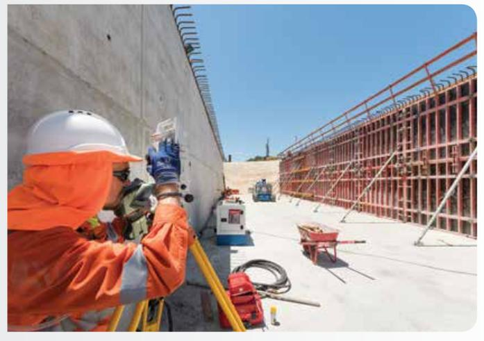
**4** To build the walls, concrete was poured between timber braces, which were removed when the concrete had hardened.
