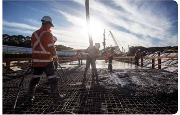
**6** The concrete roof was poured in three sections.
