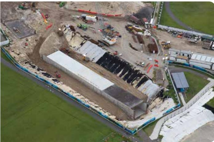
**7** This aerial view shows the new cut-and-cover tunnel complete, with back filling of soil over the tunnel underway.
