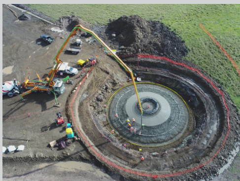
▲ Mt Gellibrand Wind Farm (under construction), VIC
